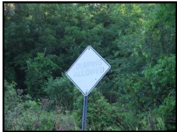
Photo 10. No dumping signage has faded and should be replaced at some NAS sites (pictured here at CE1 (Woodland Chase Trail)).
